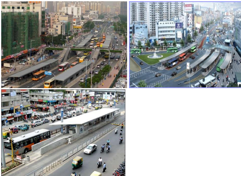
Figure 8. Contrasting approaches to pedestrian access to median-station BRT: Guangzhou (left), Seoul (middle), Ahmedabad (right). Sources: ITDP China, Cervero and Kang (2011), and author's photo.
