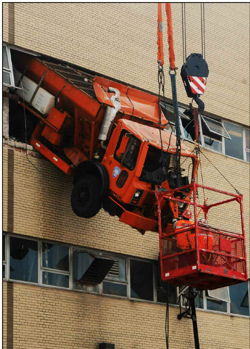
Bay Crane riggers place a sling strap around the truck to prepare it for lifting.
