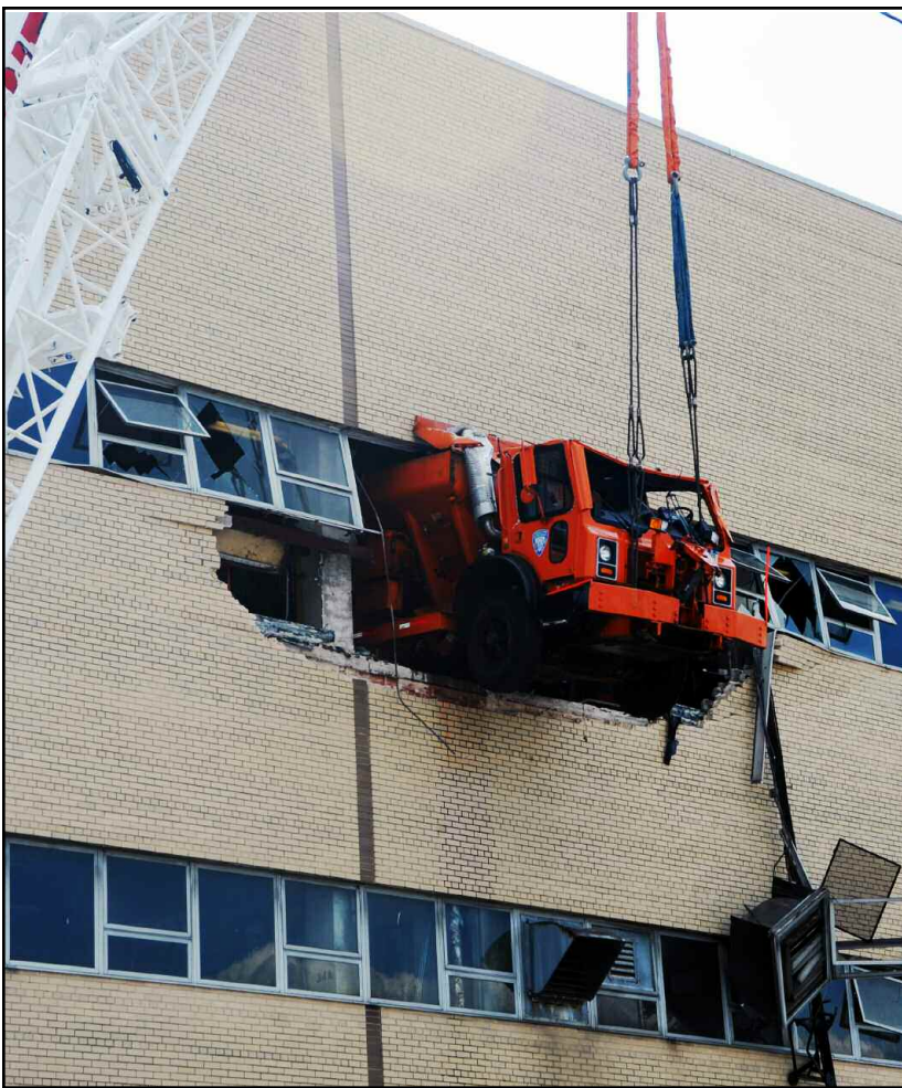
Photo #3--Crane lifts vehicle level, while griphoists pull truck into building.
